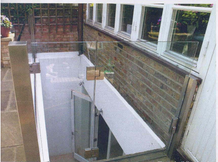
Clever building work can transform a home from underneath
